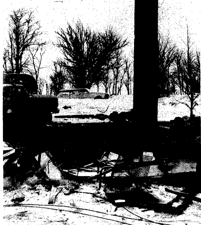
A CHIMNEY stands as mute evidence of a fire Sunday night which destroyed this house in Dixon.
